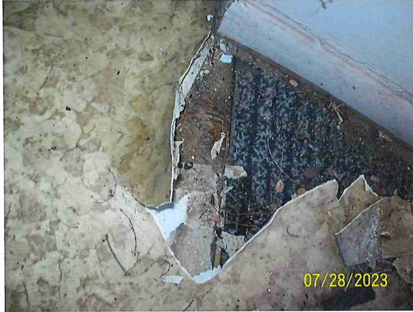
5. View of Positive Linoleum in Front Entry
