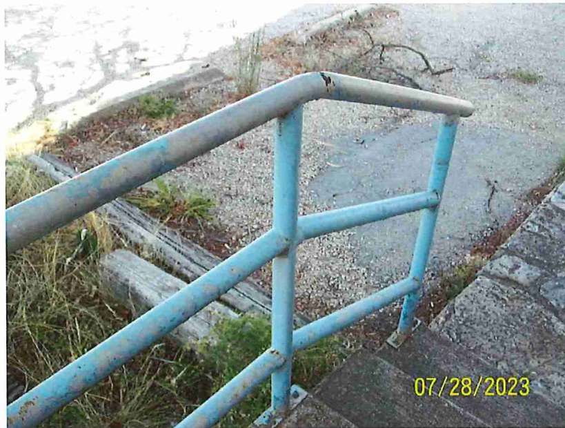
16. View of Blue Painted Railing
