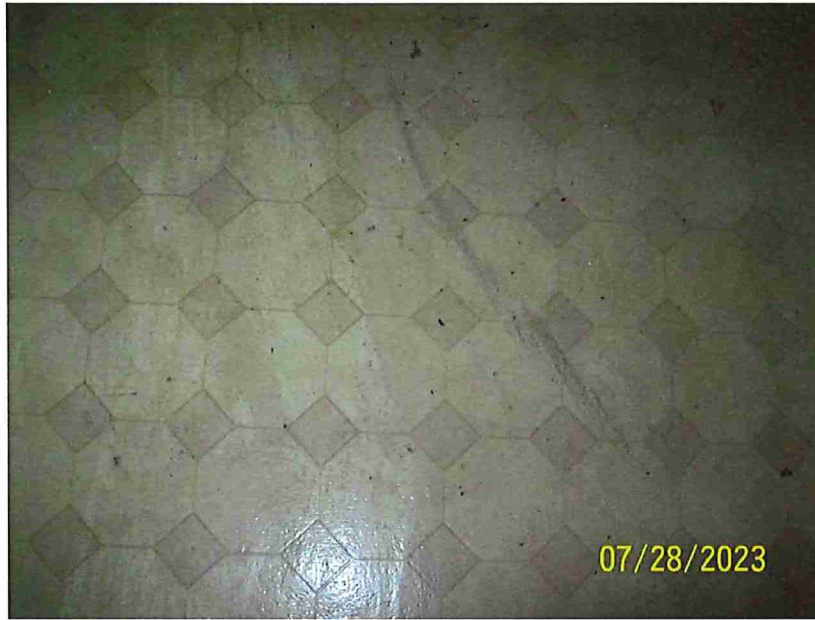
7. View of Linoleum in the Restroom
