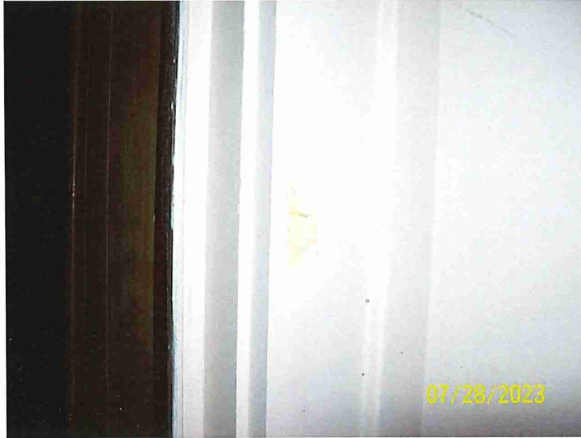
15. View of White Painted Door Frame
