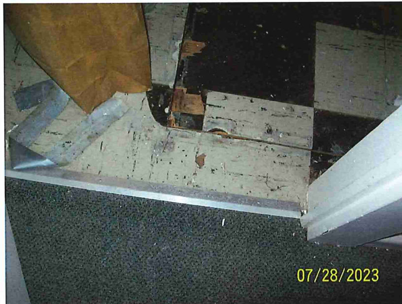
8. View of Positive Vinyl Tile with Black Felt Paper under Carpet
