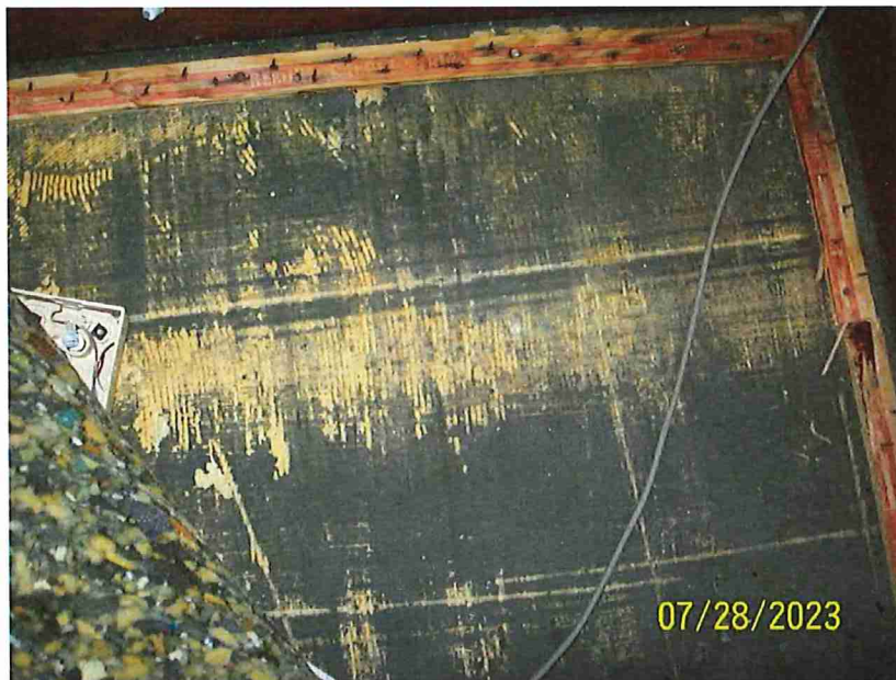
12. View of Wood Decking under Carpet
