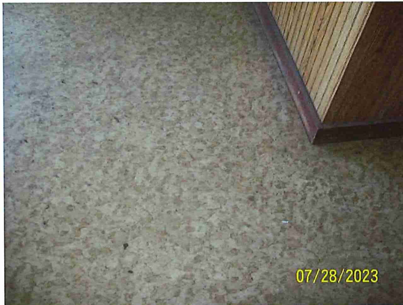
6. View of Linoleum in Restroom Hallway
