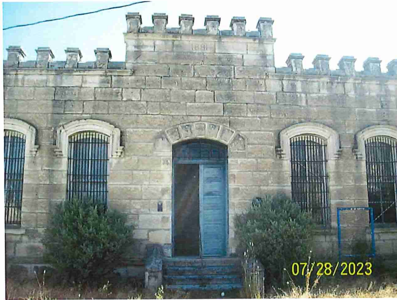
1. Exterior View of the Old County Jail located at 200 12 th Street Bandera, Texas
