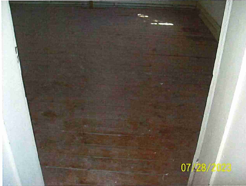
5. View of Hard Wood Flooring
