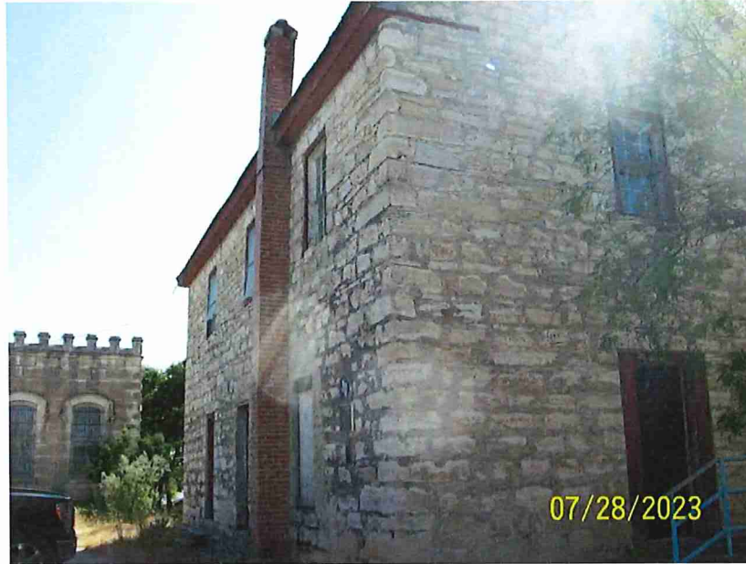
1. Exterior View of the Old County Courthouse located at 200 12 th Street Bandera, Texas
