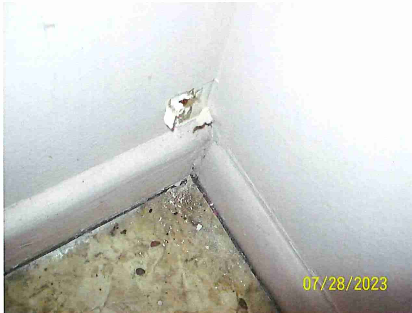
4. View of Typical Positive Wallboard with Joint Compound
