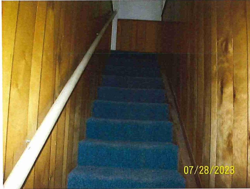
9. View of Stairs Leading to 2 nd Floor
