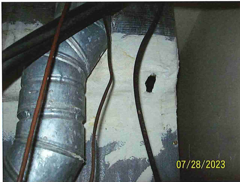
10. View of White Mastic on HVAC Unit
