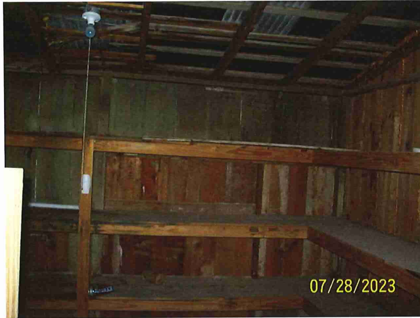
7. View of Back Shed
